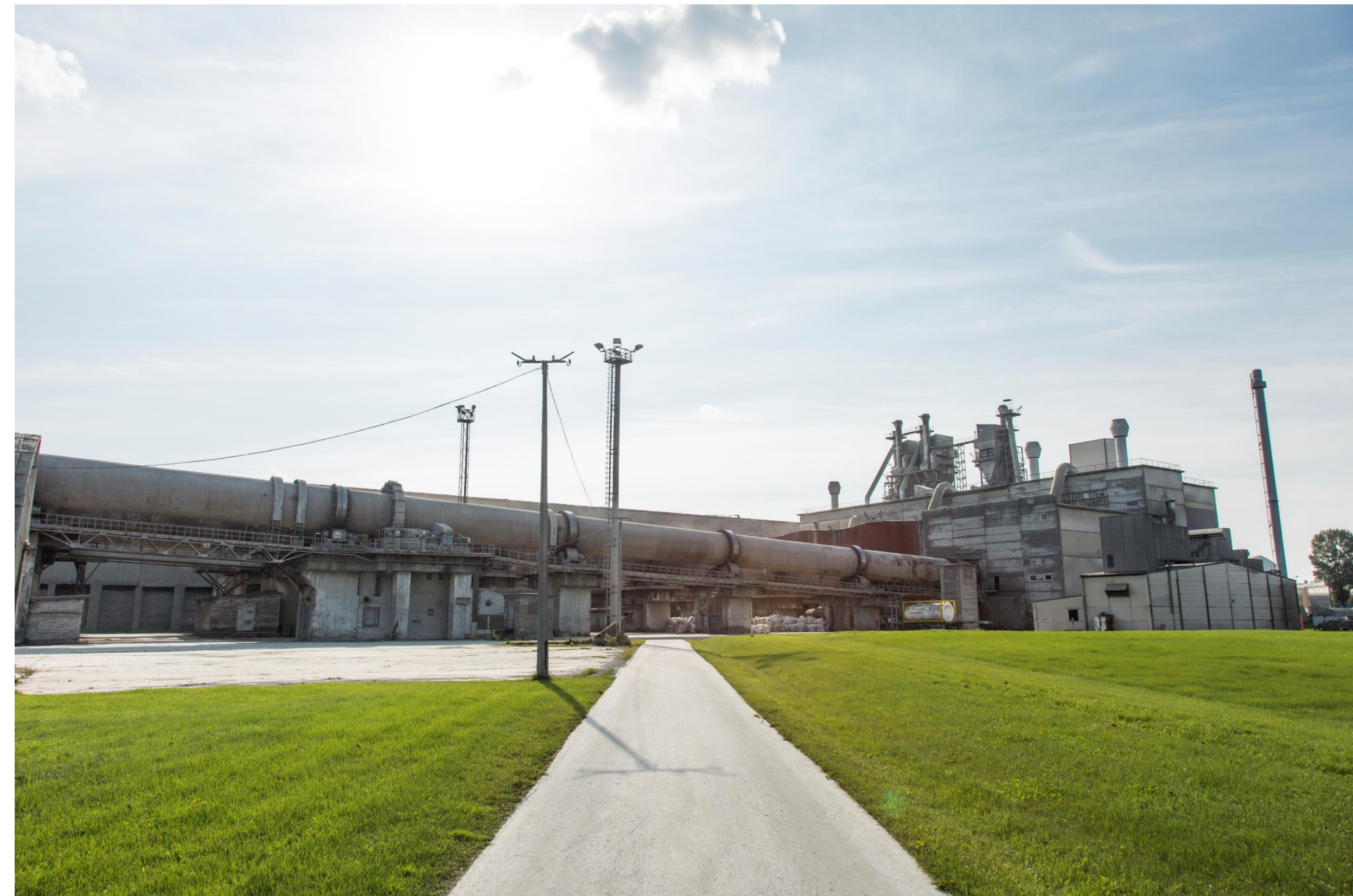
Estonia's only cement kiln was closed in 2020. It was an inefficient wet-process kiln, and the recent increase in the cost of CO 2 in the EU forced it to end operations. Upgrading to a more efficient dry-process kiln was seen as uneconomical. Photo: Kunda.
